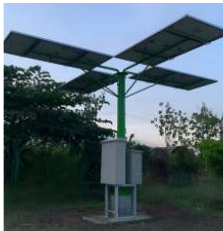
Gambar 4. Pohon panel surya (SPVT Solar Photo Voltaik Tree ).
