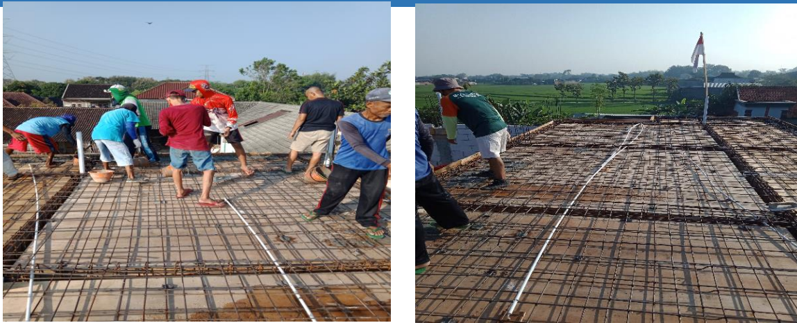
Picture 8. Thickening Of Reinforced Concrete Iron Plate
