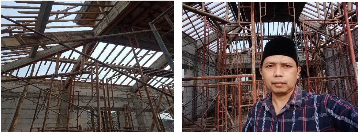
Picture 10. Roof Frame Instalation
