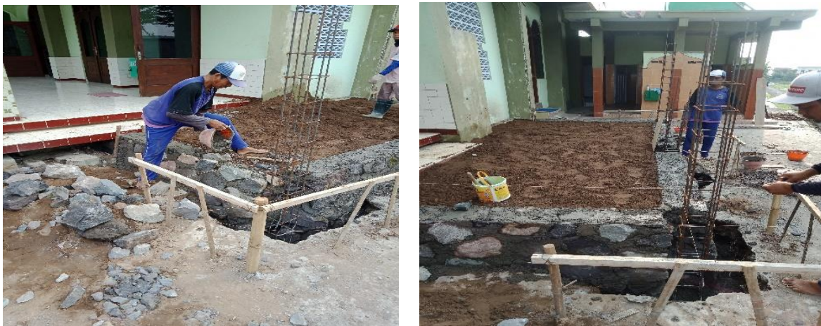
Picture 6. Concrete Food plate Foundation
